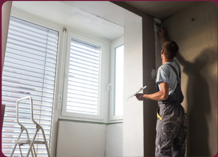
THI CÔNG SƠN PAINTING CONSTRUCTION
