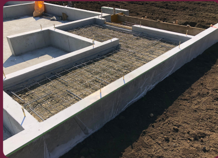
THI CÔNG MÓNG FOUNDATION CONSTRUCTION
