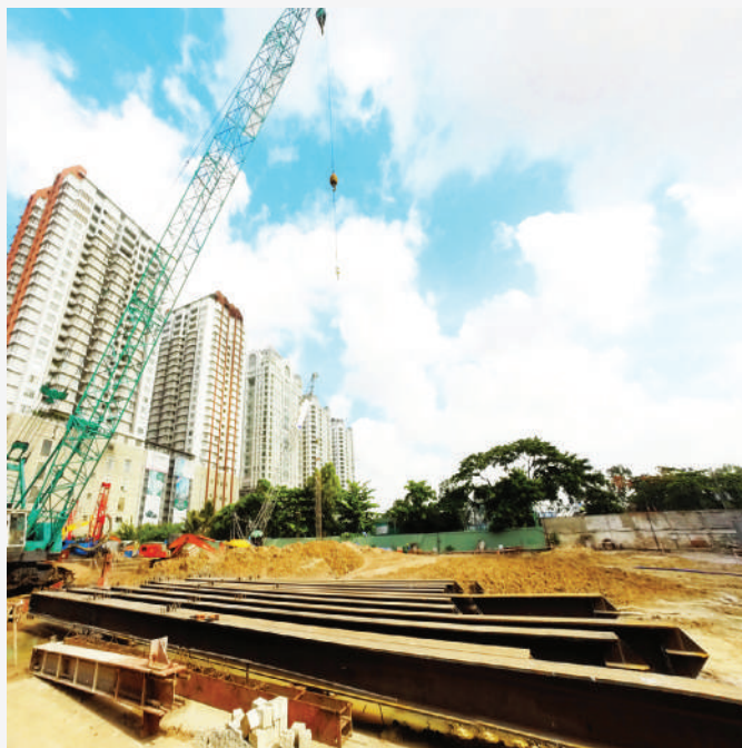
INSTALLING KINGPOST AT THE PARK AVENUE CONSTRUCTION
