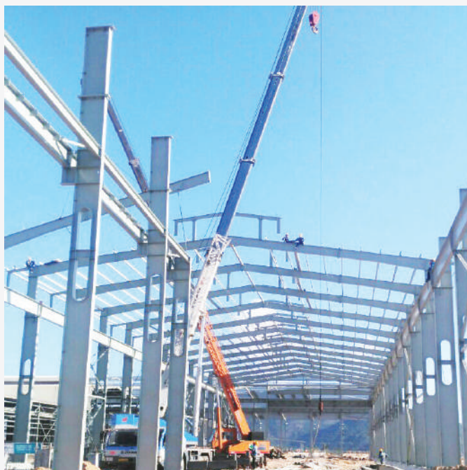
INSTALLING FRAMING RAFTERS AT HOA SEN NHON HOI - BINH DINH FACTORY
