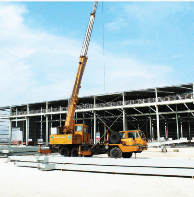
INSTALLING FRAMING RAFTERS AT HOA SEN HA NAM FACTORY
