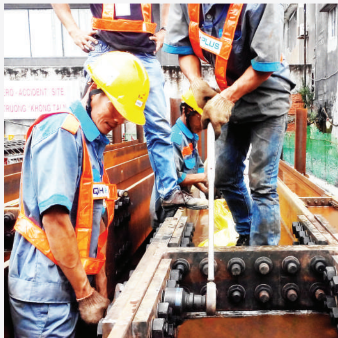
INSTALLING KINGPOST AT ETOWN CENTRAL CONSTRUCTION
