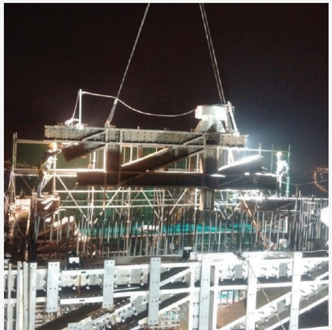
INSTALLING STEEL CORE SYSTEM AT VINHOMES LANDMARK 81 FLOORS
