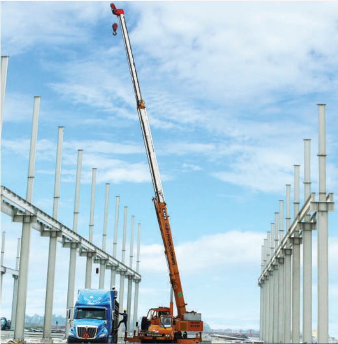
INSTALLING STEEL BUILDING FRAME AT HOA SEN HA NAM FACTORY
