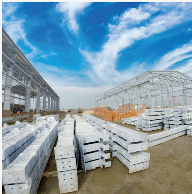
INSTALLING PRE-ENGINEERED BUILDING AT BA SON SHIP YARD
