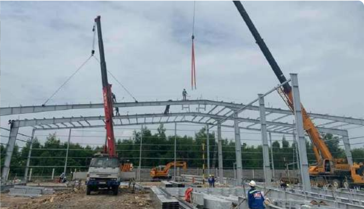
6 NHÀ MÁY CITY FOCUS LIGHTING CITY FOCUS LIGHTING工厂
