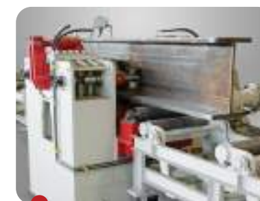
Nắn dầm | Straightening beams
