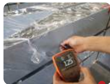
Kiểm Tra Sơn | Inspection Painting
